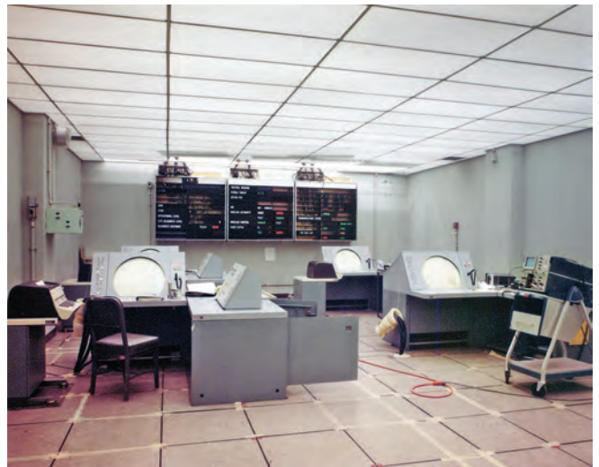
Historic view of the BMDOC showing the four consoles during installation. The panels on the rear wall showed system status. Provided by Clint Esciklsen
